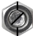
(Bolt is loose)
